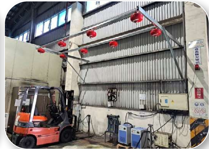
Suspended fire extinguishers have been installed above the forklift charging zones
