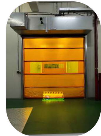
Sensor Projection Lights Above Fire-Rated Shutters
