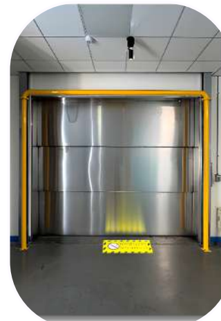
Sensor Projection Lights Above Fire-Rated Shutters
