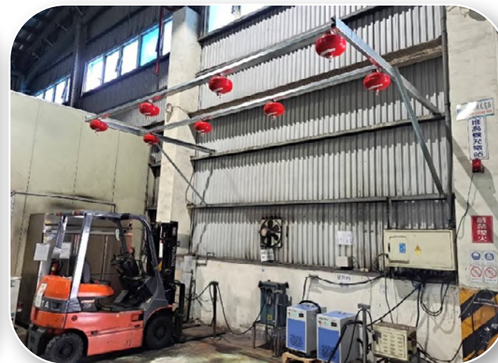
Suspended fire extinguishers have been installed above the forklift charging zones
