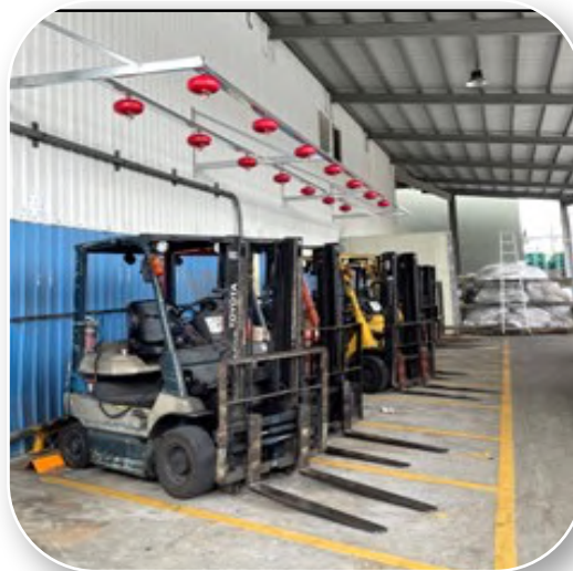
Suspended fire extinguishers have been installed above the forklift charging zones
